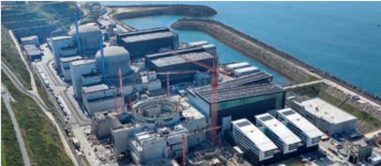
Flamenville construction site. Image courtesy of EDF. © Copyright EDF – Alexis MORIN.
