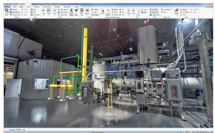
Laser scan data integrated into the 3D view
