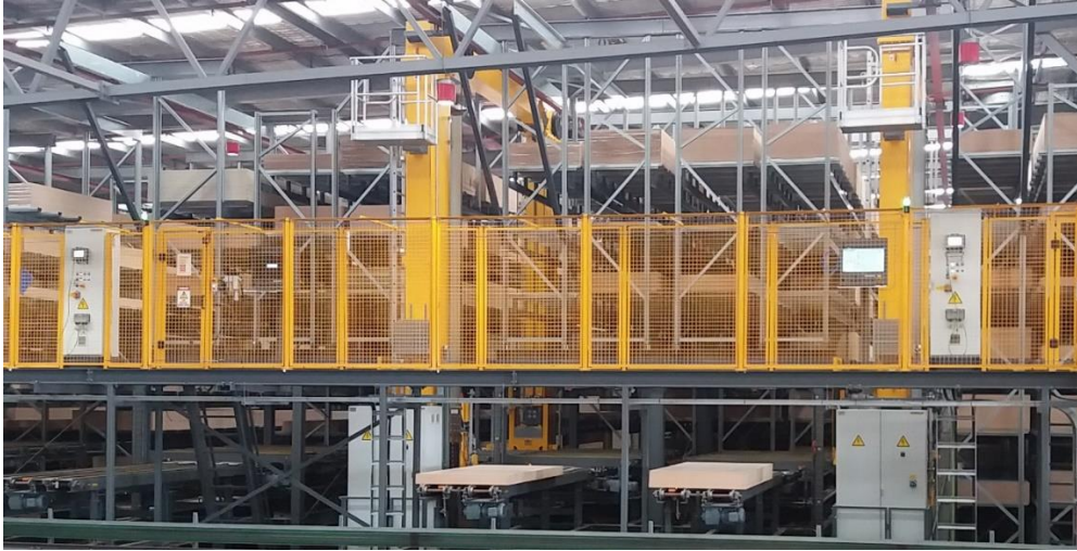
Figure 3 – ASRS Cranes in the main warehouse storage section
