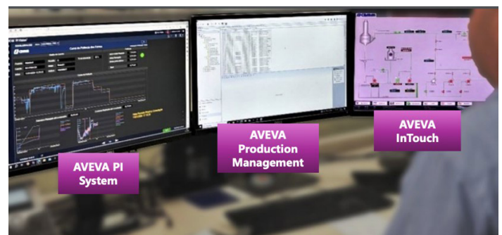
With three existing AVEVA solutions, CBMM and Stefanini developed one integrated system to implement, standardize, and manage power curves.
