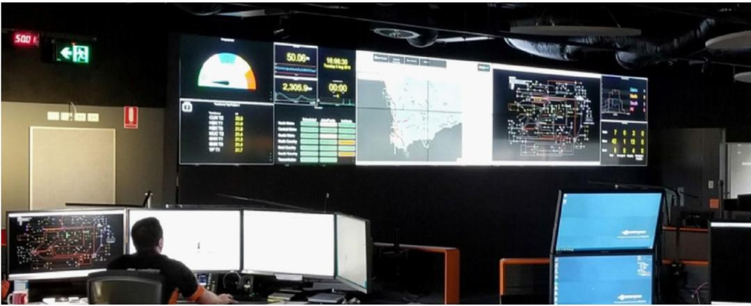
Video walls are installed around Western Power's Network Operations Centre, with PI Vision displays providing real-time operational awareness across the entire transmission network.
