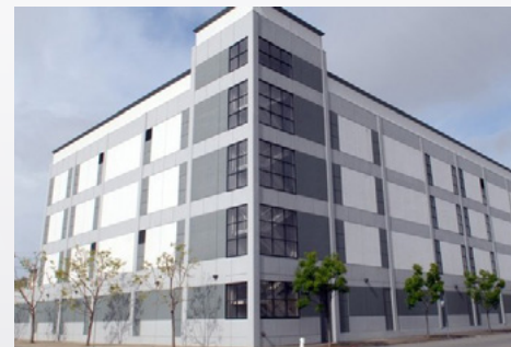
Digital Realty's Oakland data center
